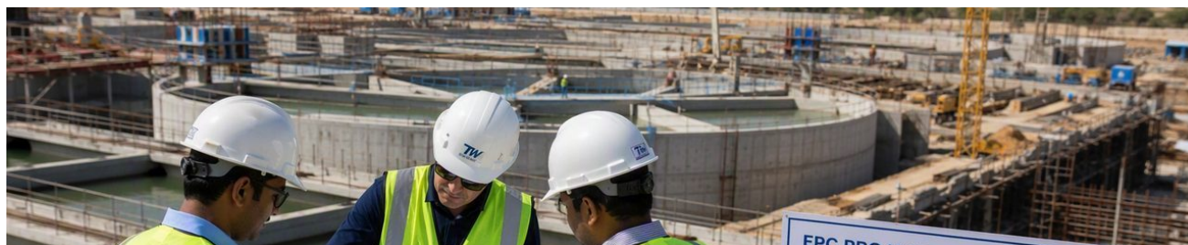
Figure 1 — EPC delivery in progress — process design, procurement and construction under one accountable P.Eng.
